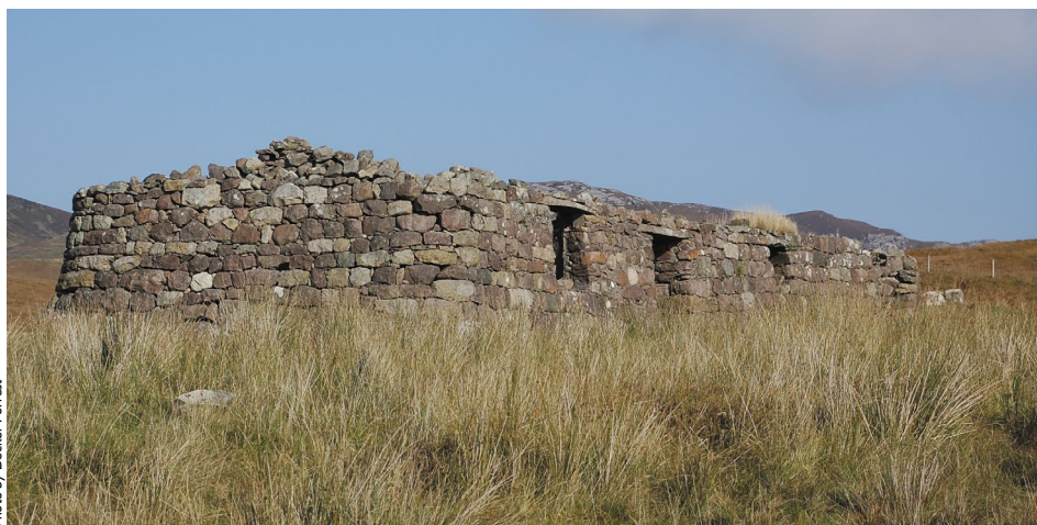
The Piper's House showing the exceptional drystone walling construction.
